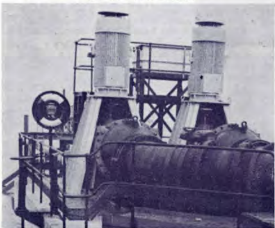
The electric pumps used to transfer water from the River Mersey to the Manchester Ship Canal to compensate for the water taken out of the Canal by Ince Power Station
