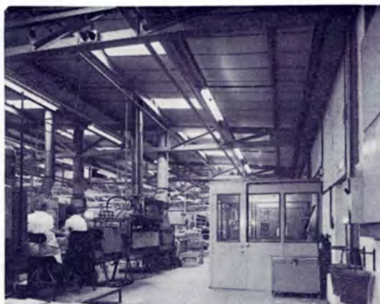
△ Lighting and power in the engineering works of Francis Industries at Wrexham
