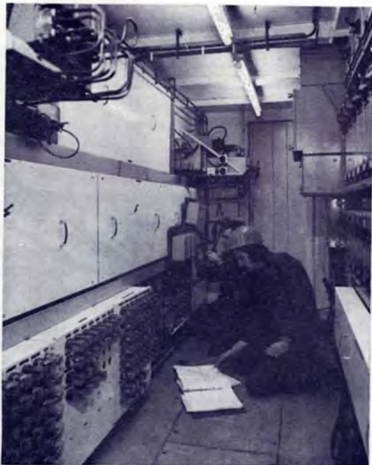
MANWEB electricians wiring a control panel at Five Fords sewage works at Marchwiell near Wrexham, part of a handy installation contract worth £30,000. We also have a maintenance contract from the Welsh National Water Development Authority bringing in £11,500 a year.
